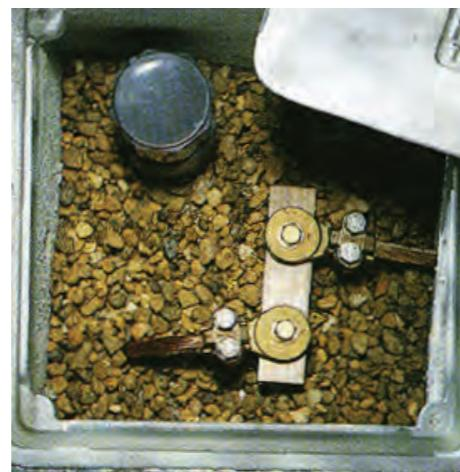
Fig. 14 – Registry system of grounding installation.
